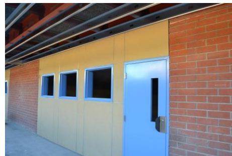
Finished Exterior Plaster Building 2
